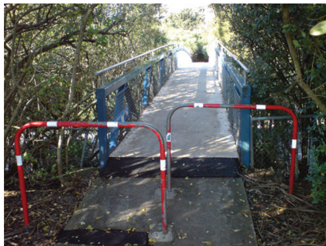
Barriers preventing wheelchair access across an otherwise accessible bridge in Auckland City, New Zealand. Photograph by Ingolfson, Wikimedia Commons.
